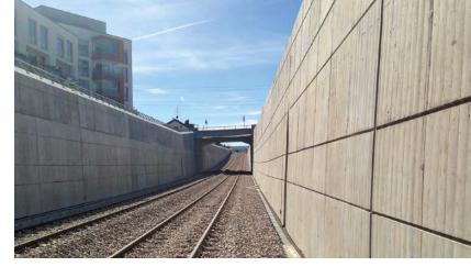
After more than a year of construction, the earthworks as well as the concrete and steel construction work have now been completed. Only the modelling of the terrain around the structures and the lanes still need to be finalised. The train route, which is currently closed, is expected to open by December. Until then the Schönbuchbahn project will also be finalised, offering road users a new and collision-free crossing.
